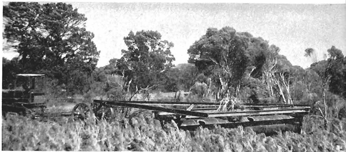
Clearing and rolling scrub in the Keith area.
