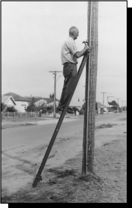
Installing male annihilation blocks.
